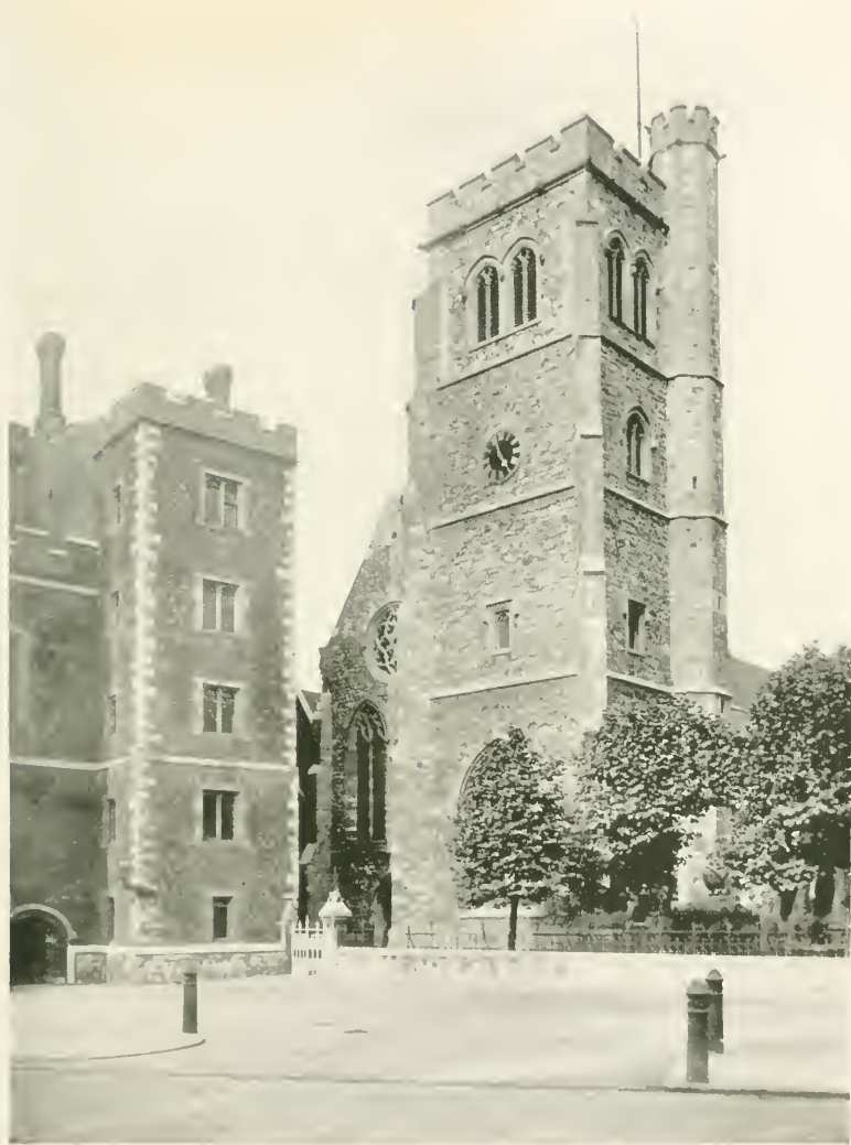
LAMBETH CHURCH AND PALACE GATE
